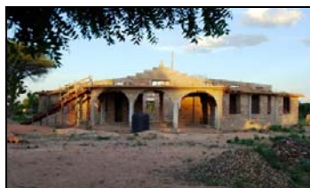
The progress of the Mwitikira church construction.
