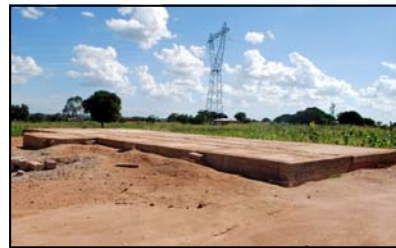
The foundation of the Nala library.
